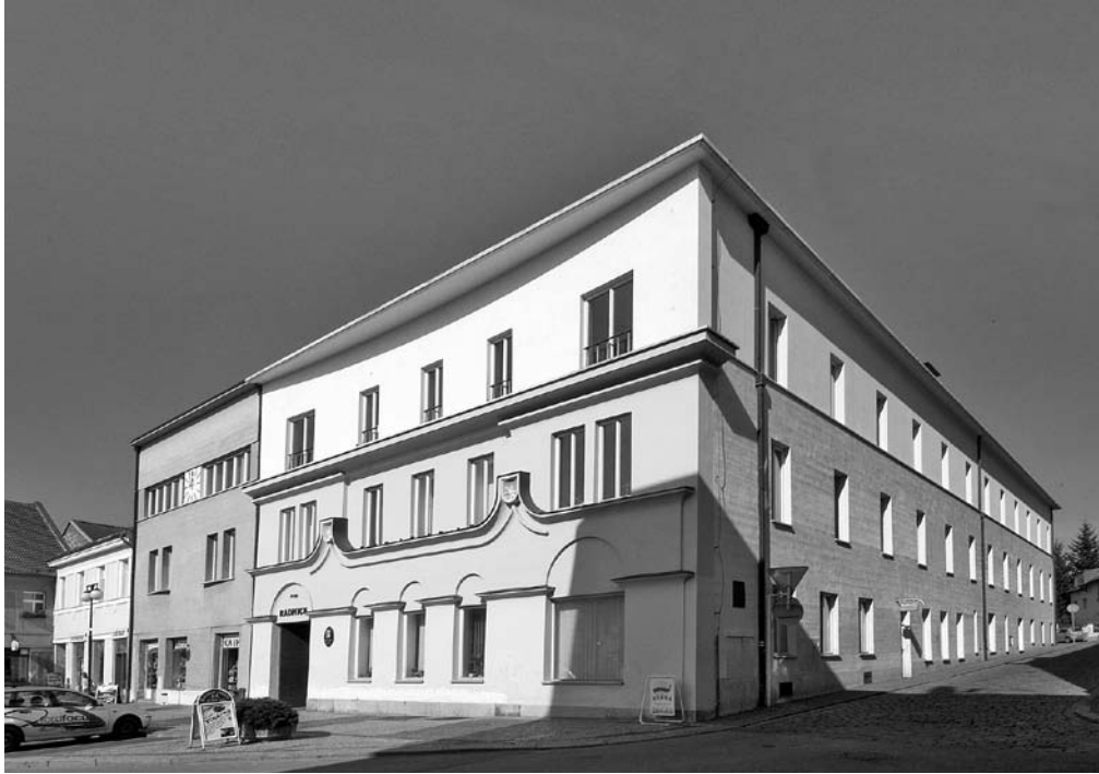
Architecture for reborn democracy that preserves memory and identity. Benešov, alteration and expansion of the City Hall, designed by Josef Pleskot, Radek Lampa, Vladimír Krajíc and Jana Vodičková, 1993–1995
