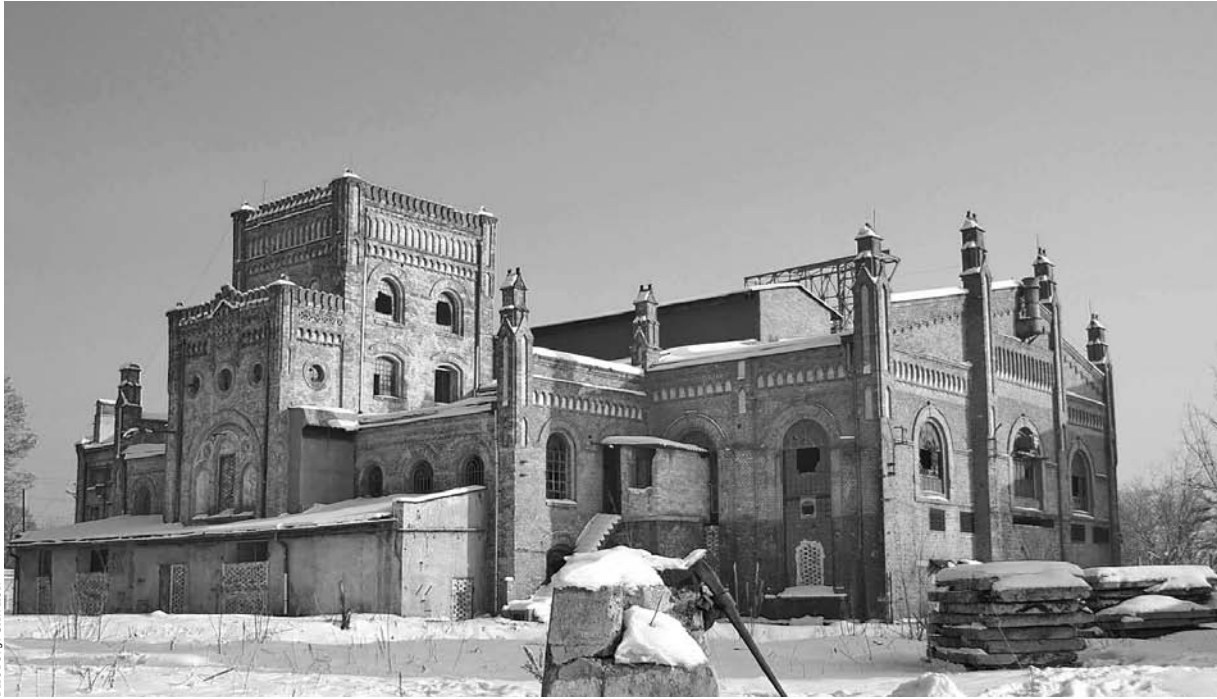
Katowice, buildings of the former Katowice Coal Mine, power plant of the Bartosz shaft
