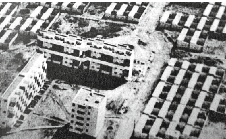
SHADRACH WOODS COLLECTION, DRAWINGS AND ARCHIVES, AVERY ARCHITECTURAL AND FINE ARTS LIBRARY, COLUMBIA UNIVERSITY/COURTESY OF NAI PUBLISHERS
