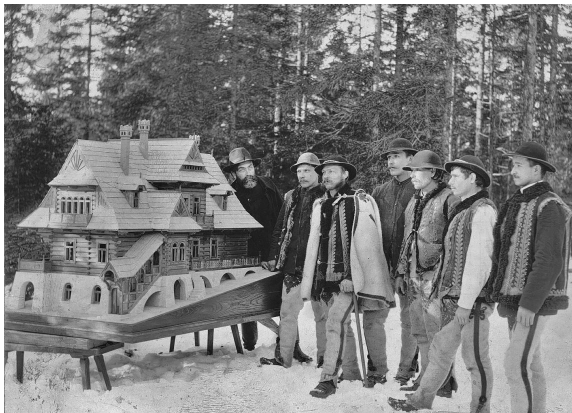
Stanisław Witkiewicz and the contractors of the House under the Firs (Dom Pod Jedlami) with its model, December 1899
